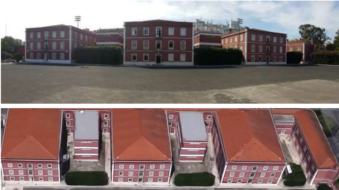
Figure 2 Barracks building in analysis
